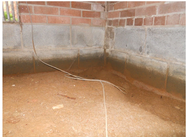
Water staining/ trench at front left corner
