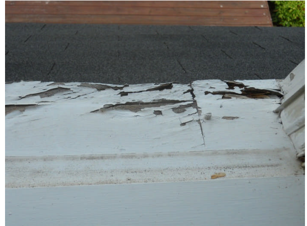
Damaged window stool on upstairs bay window
