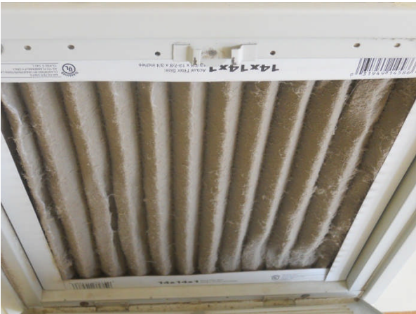
Air filter needs changing
