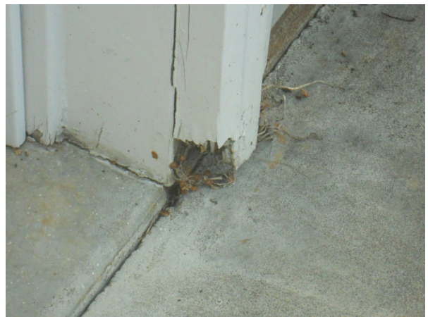
Damaged wood trim on garage door
