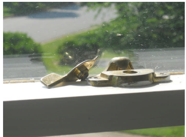
Broken window lock
