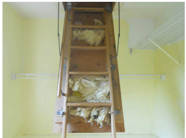
Attic pull down steps need new batt insulation
