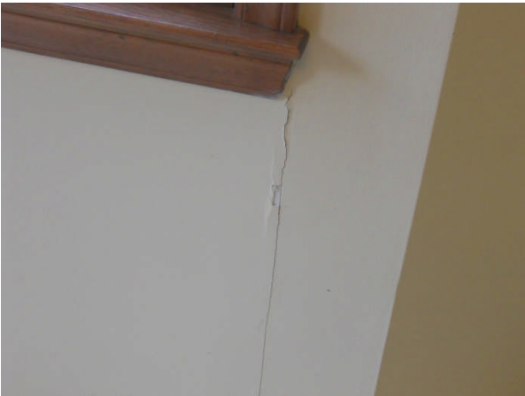
Crack under rear living room bay window
