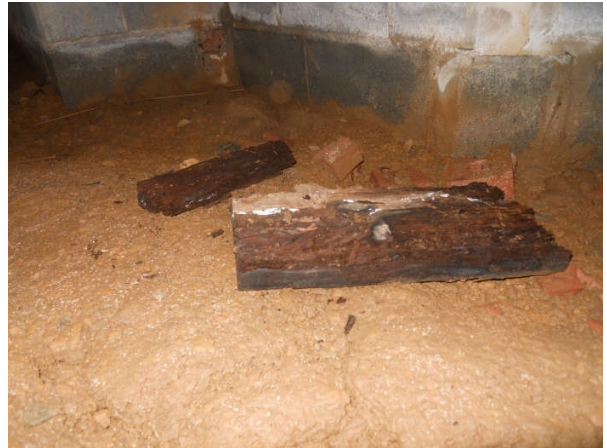
Wood debris in the crawlspace
