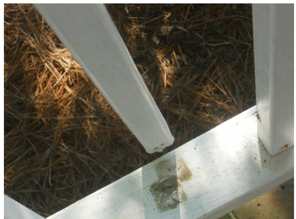
Loose pickets on front handrail
