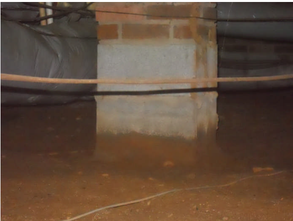
Water staining on piers
