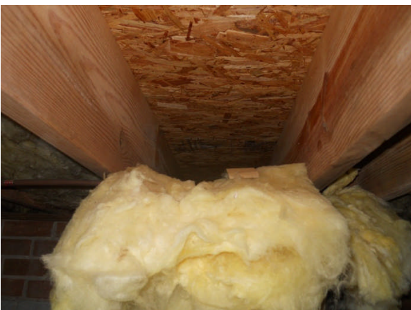
Fallen/ missing insulation
