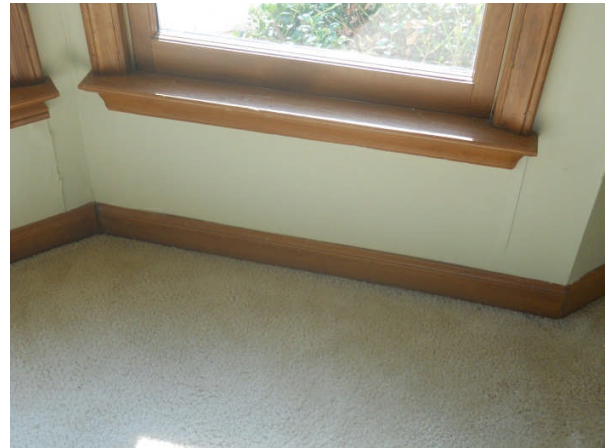
Crack under front downstairs bay window
