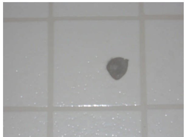
Damaged master bath vinyl flooring
