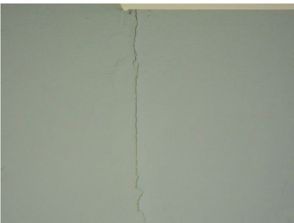
Crack under upstairs bay window
