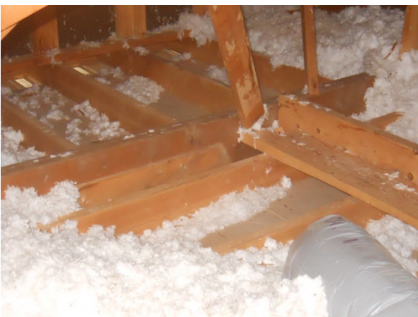
Missing insulation in attic
