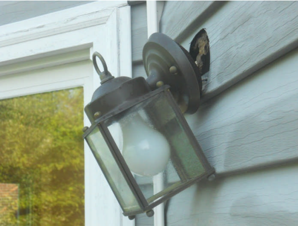
Rear deck light is not secured to the house
