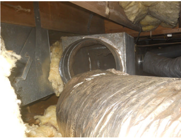
Disconnected air duct in crawlspace
