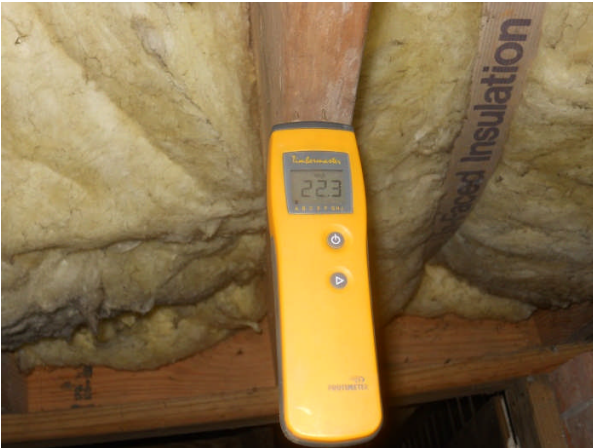
Moisture reading high in floor joists
