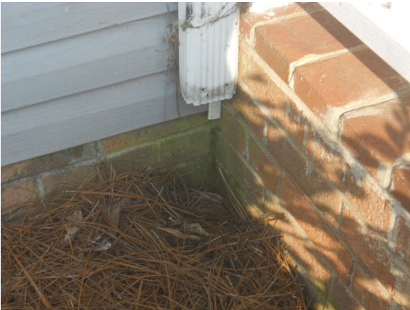
Missing elbow/ drain pipe at downspout
