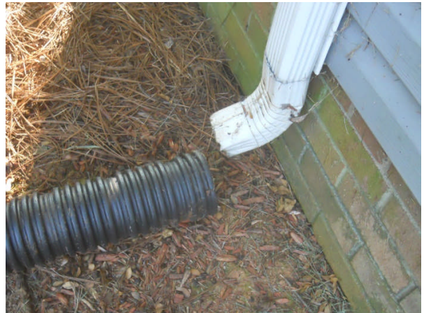
Downspout not connected to drain pipe
