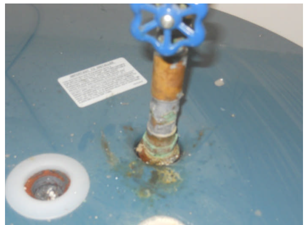
Water heater handle has some water at it
