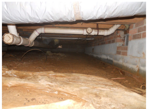
Missing vapor barrier
