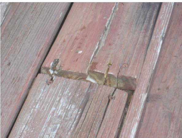
Loose decking boards
