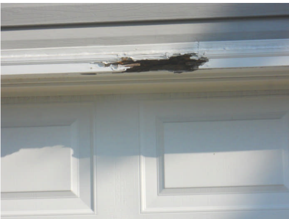
Damaged wood trim on garage door
