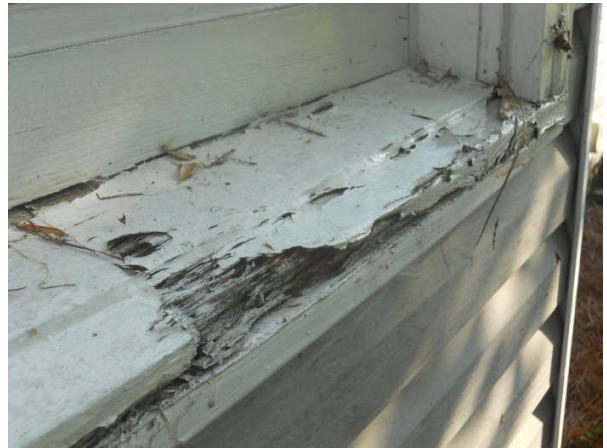
Damaged window stool on left side window
