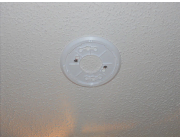
Missing smoke detector downstairs
