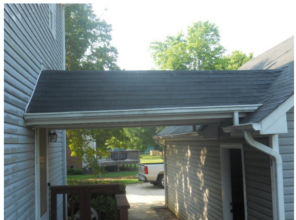
Breezeway gutter slopes the wrong way
