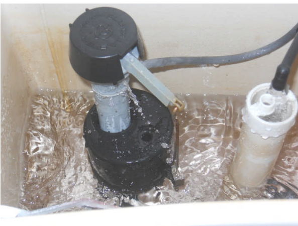
Flush valve kit in toilet need changing
