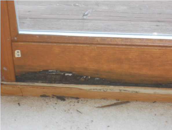
Damaged living room door
